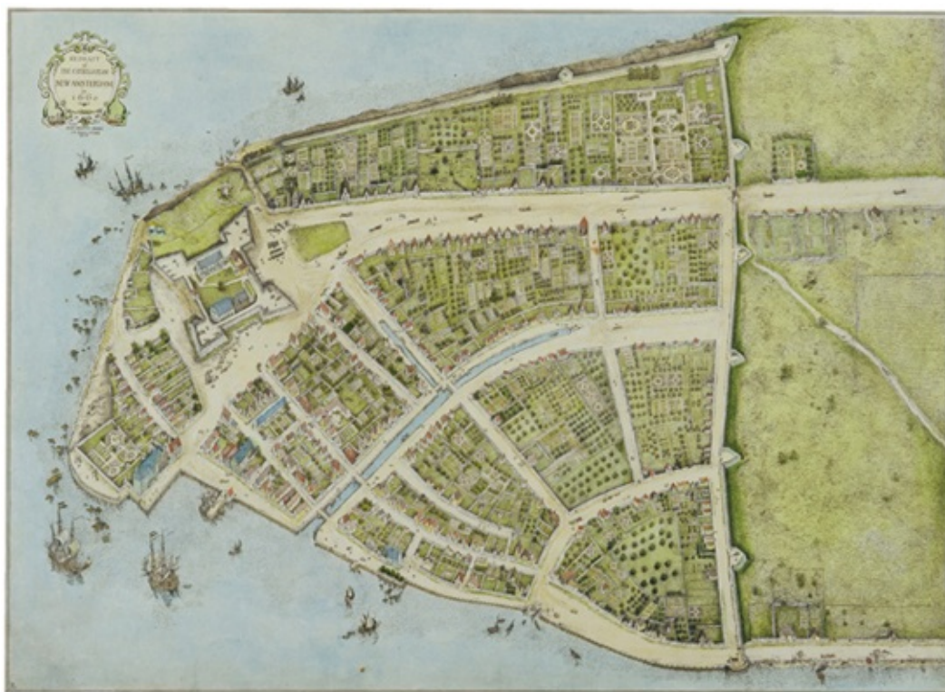
39. New Amsterdam in 1660, at the tip of Manhattan Island. The settlement's protective wall is today paved over by Wall Street.
